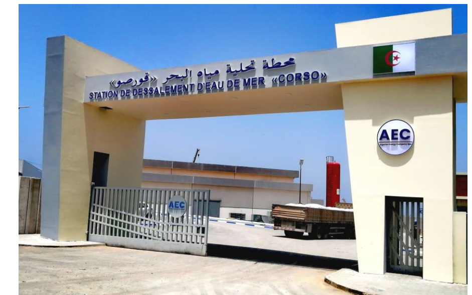
El Marsa with a capacity of 60,000 m 3 /day
